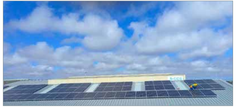
Solar array underway at Pienaar Bros, Paarden Eiland.
