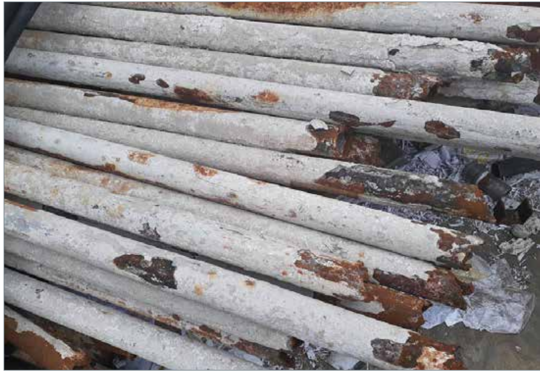
Damaged boiler tubes.
