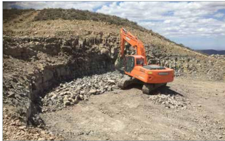
Wind turbine foundation excavation being undertaken
