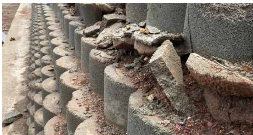
No drainage, no supervision, no reinforced concrete infill as specified.
