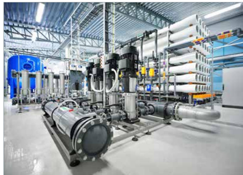
Water treatment plant including reverse osmosis module.
