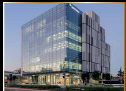
Cape Concrete Work's precast concrete panels integrate seamlessly with the glazed facades of the recently completed Investec building at Cape Town's V&A Waterfront.
