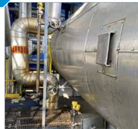
VEGAFLEX 81 guided wave radar sensors measure the separation layers in the 3-phase separator.
